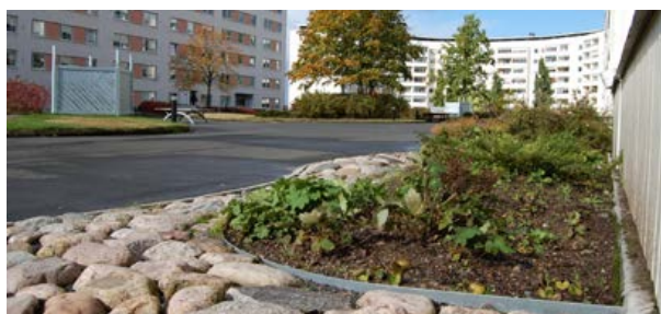
Steellight monterat i Jönköping.
